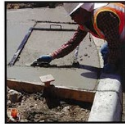
3. Remove 3/4" of concrete
