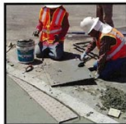
5. Apply 1/8" bonding mortar
