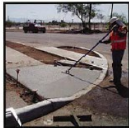
1. Finish concrete to proper grade
