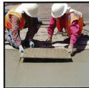
6. Install into 'fresh' concrete
