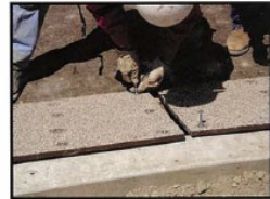
4. Insert the bolts into nuts on back of tiles
